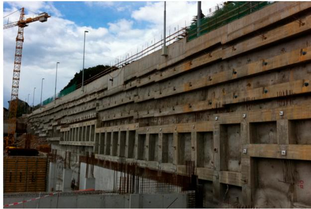
Figure 1. An example of the installed rock bolt system.
