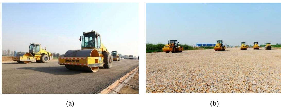
**Figure 18.** Upgraded recycled aggregates used in highway construction: (a) Base constructed using purified MRA; (b) Sub-base constructed by brick mixed MRA.
