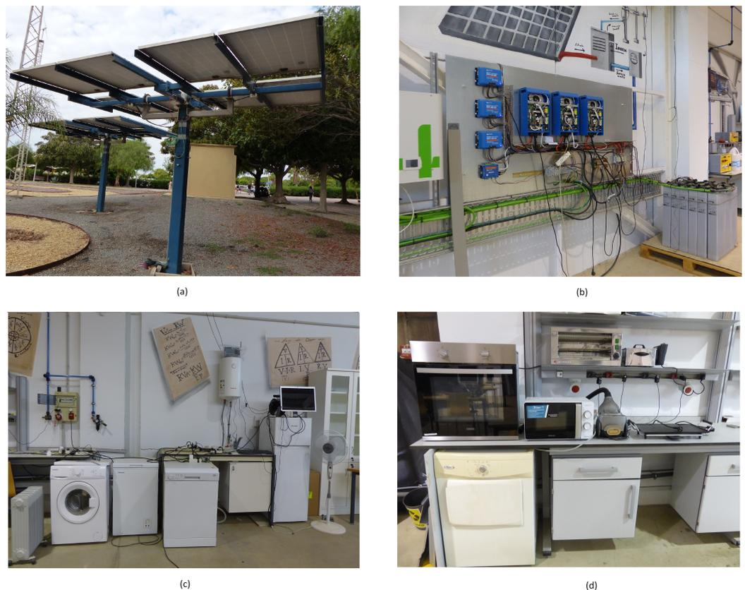
**Figure 2.** (a) Photovoltaic solar trackers; (b) power electronics and storage systems; (c,d) loads (home appliances).
