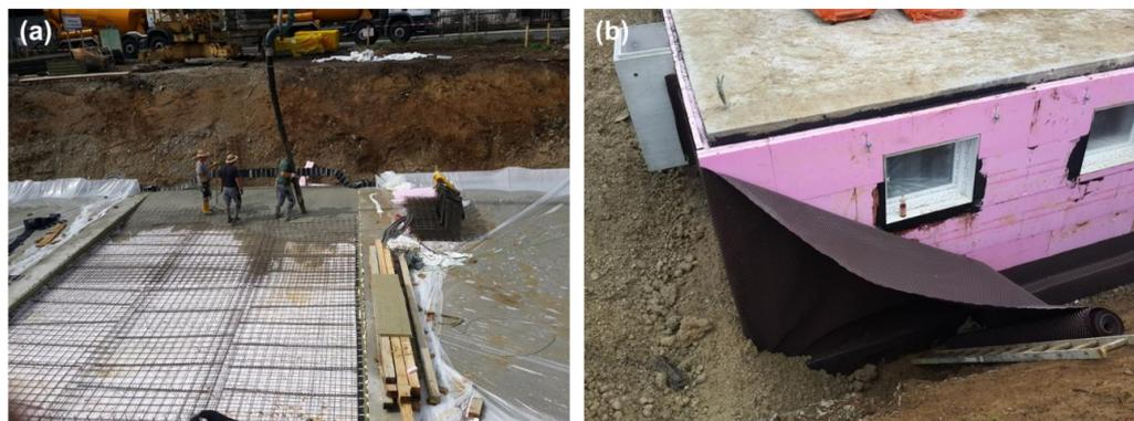
**Figure 7.** Measures to prevent rising damp on a construction site in Germany: (a) measures for a lower ground floor, (b) measures for basement walls.
