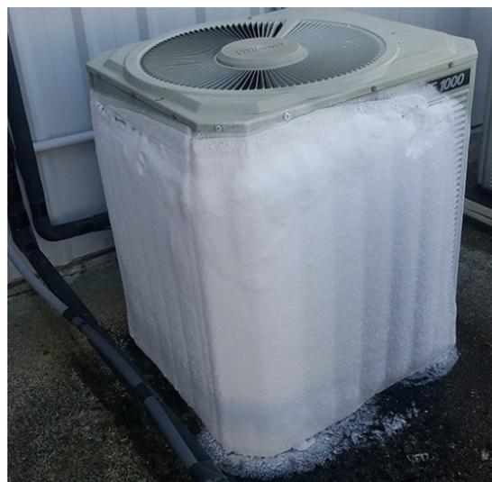
**Figure 4.** Frost fully blocking heat pump. Reproduced with permission from [10], Elsevier, 2022.
