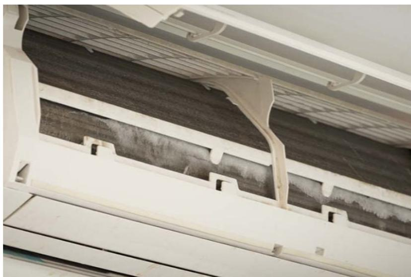
**Figure 5.** Frost fully blocking air conditioning system. Reproduced with permission from [11], Elsevier, 2022.
