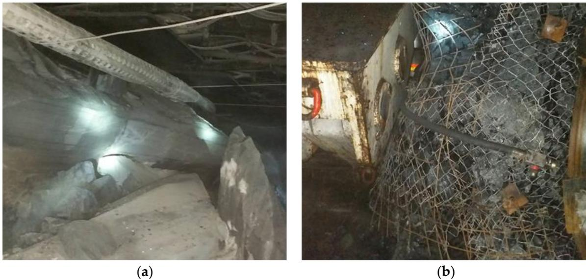
**Figure 2.** 31,105 ground pressure behavior during final mining retracement of working face: (a) roof fall of working face; (b) the retracement roadway is severely deformed.
