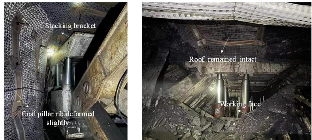
Figure 18. Illustration after the evacuation channel is completed.
