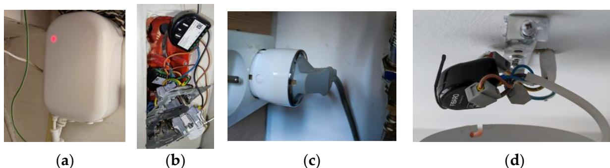
**Figure 6.** Photographs of sample installed measurement systems: (a) AEOTEC meter installed in the building’s switchboard; (b) Fibaro switch in flush-mounted socket; (c) Fibaro wall-plug; (d) Fibaro switch in the housing of the ceiling lamp. Source: author’s development.
