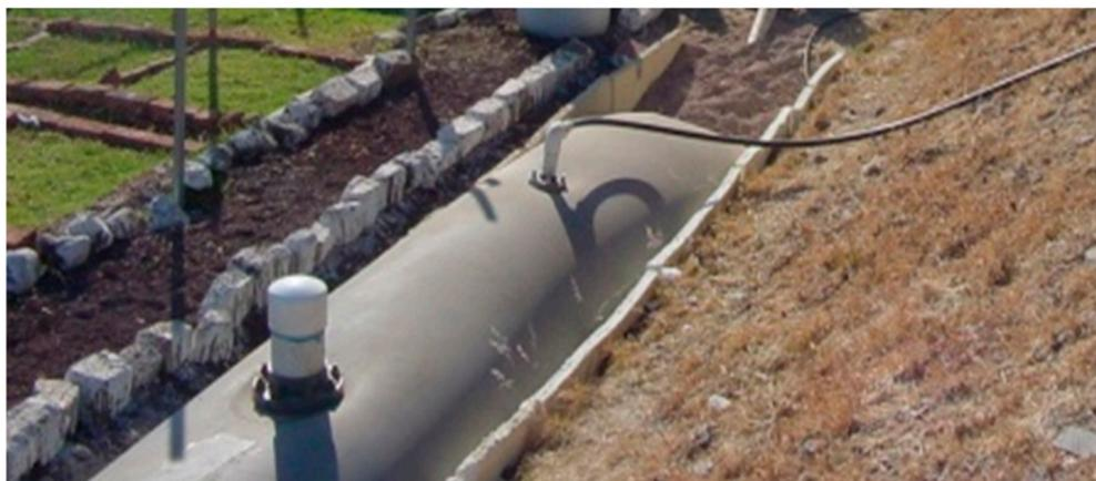
**Figure 3.** Picture of the plug-flow anaerobic digester (9 m<sup>3</sup>) for testing system parameters.
