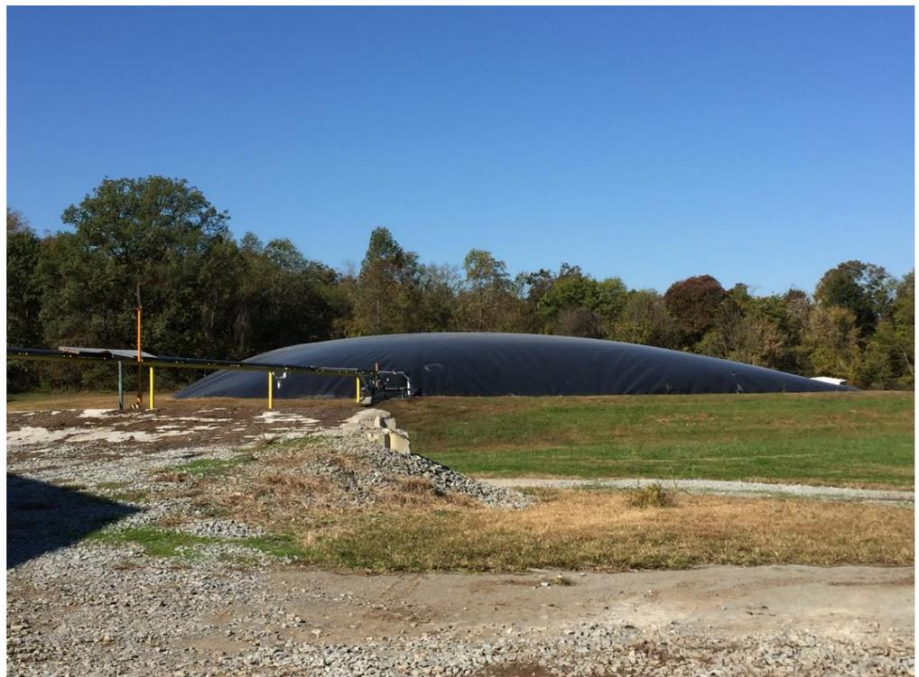
**Figure 2.** Picture of the lagoon (pond) anaerobic digester (57 million liters).
