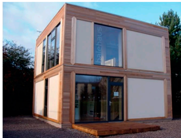
Figure 4. BaleHaus, University of Bath: Straw load-bearing walls [43].
