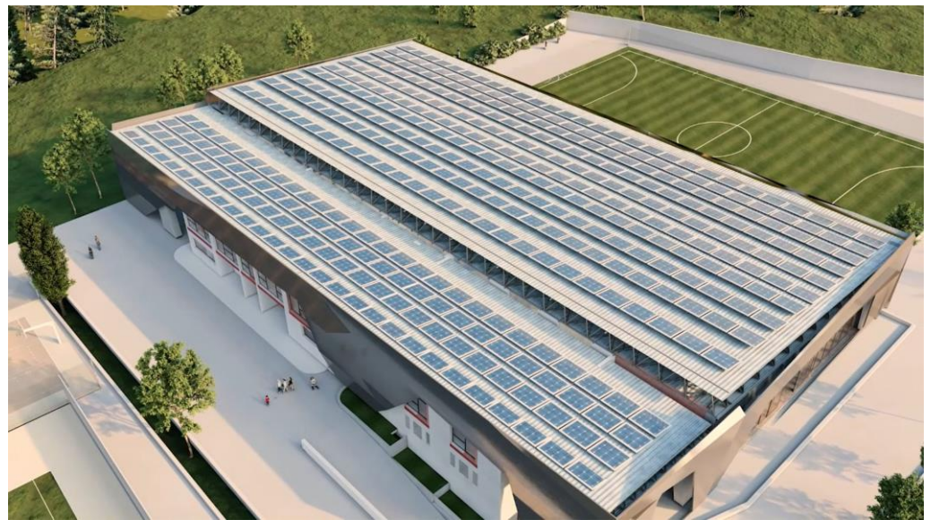
Figure 26. A 3D representation of the photovoltaic plant on the roof of the swimming pools' new enclosure.
