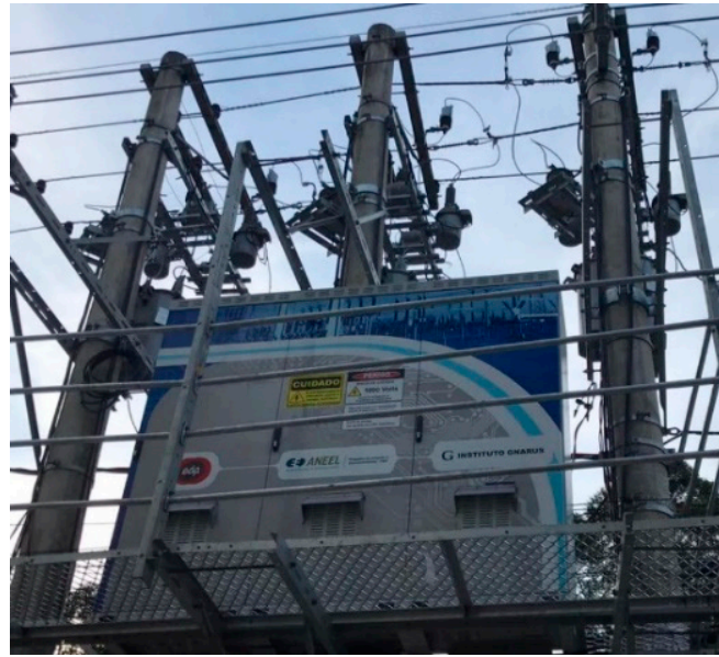
Figure 10. Developed three-phase series converter in outdoor installation—13.8 kV field test.
