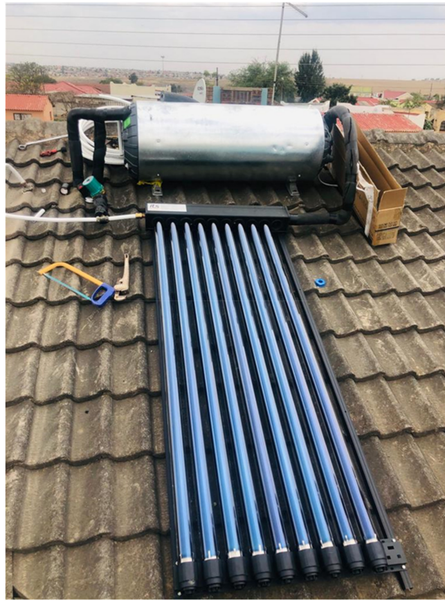
Figure 3. The installation of the SWH in the experimental residence in Dimbaza.
