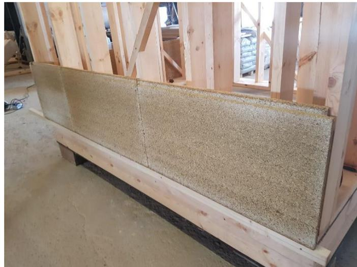
**Figure 9.** MOC biocomposite boards during construction of timber frame testing facility.
