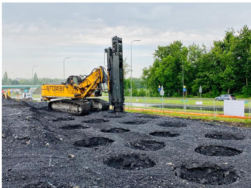
**Figure 23.** RIC impulse compactor in operation (Photo by P. Dobrzycki).
