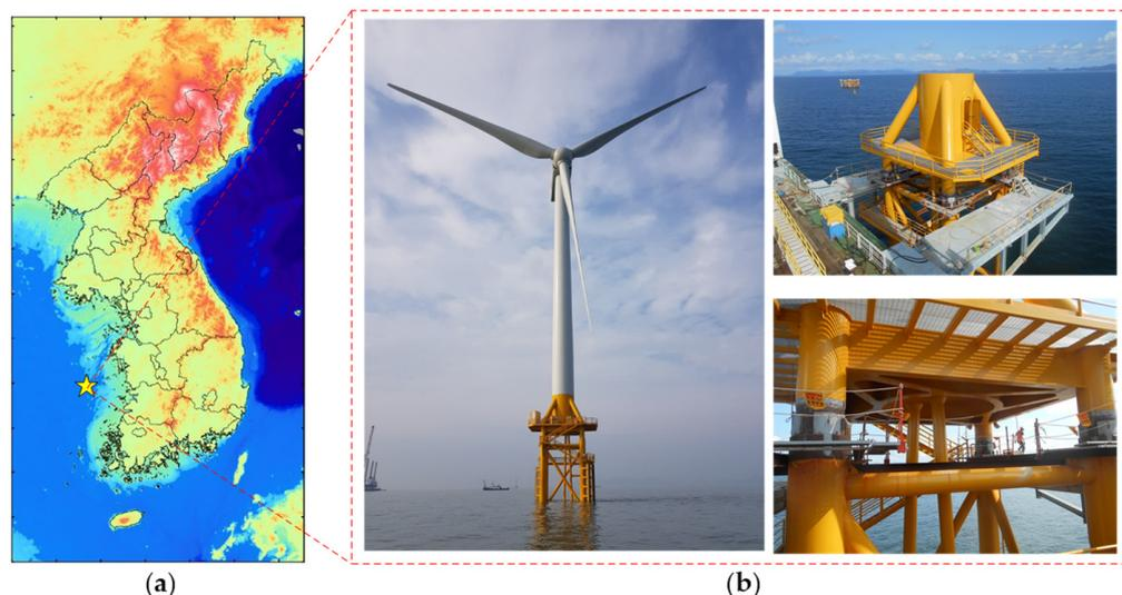
**Figure 1.** A 3MW offshore wind turbine selected for the study: (a) Site location; (b) A 3MW jacket substructure.
