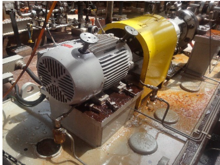
Figure 3. Industrial electric motor driving a wastewater pump.
