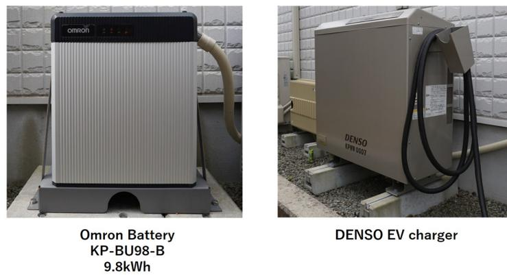
Figure 3. Hardware installed at participant homes.
