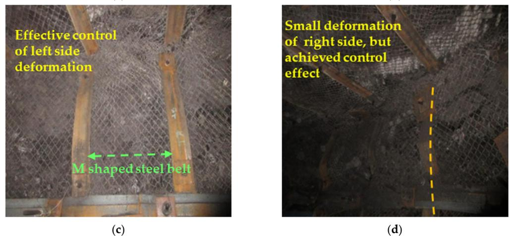
**Figure 22.** Application effect of the full-stress anchoring plan of bolts. (a) Roof control effect; (b) side-angle control effect; (c) left-side control effect; (d) right-side control effect.
