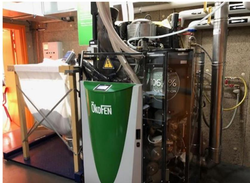
Figure 5. Micro-CHP unit installed in laboratory@ Paris Nanterre University.
