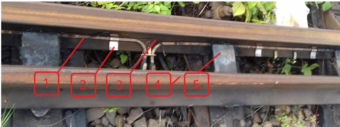
**Figure 2.** Built-in flat-oval resistance heaters (1) mounted with special holders (2) to the foot of the stock rail (3); (4)—switch rail, (5)—plates.
