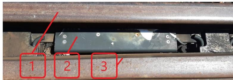
**Figure 4.** IH device heating part (2) mounted between the stock rail (1) and the switch rail (3).
