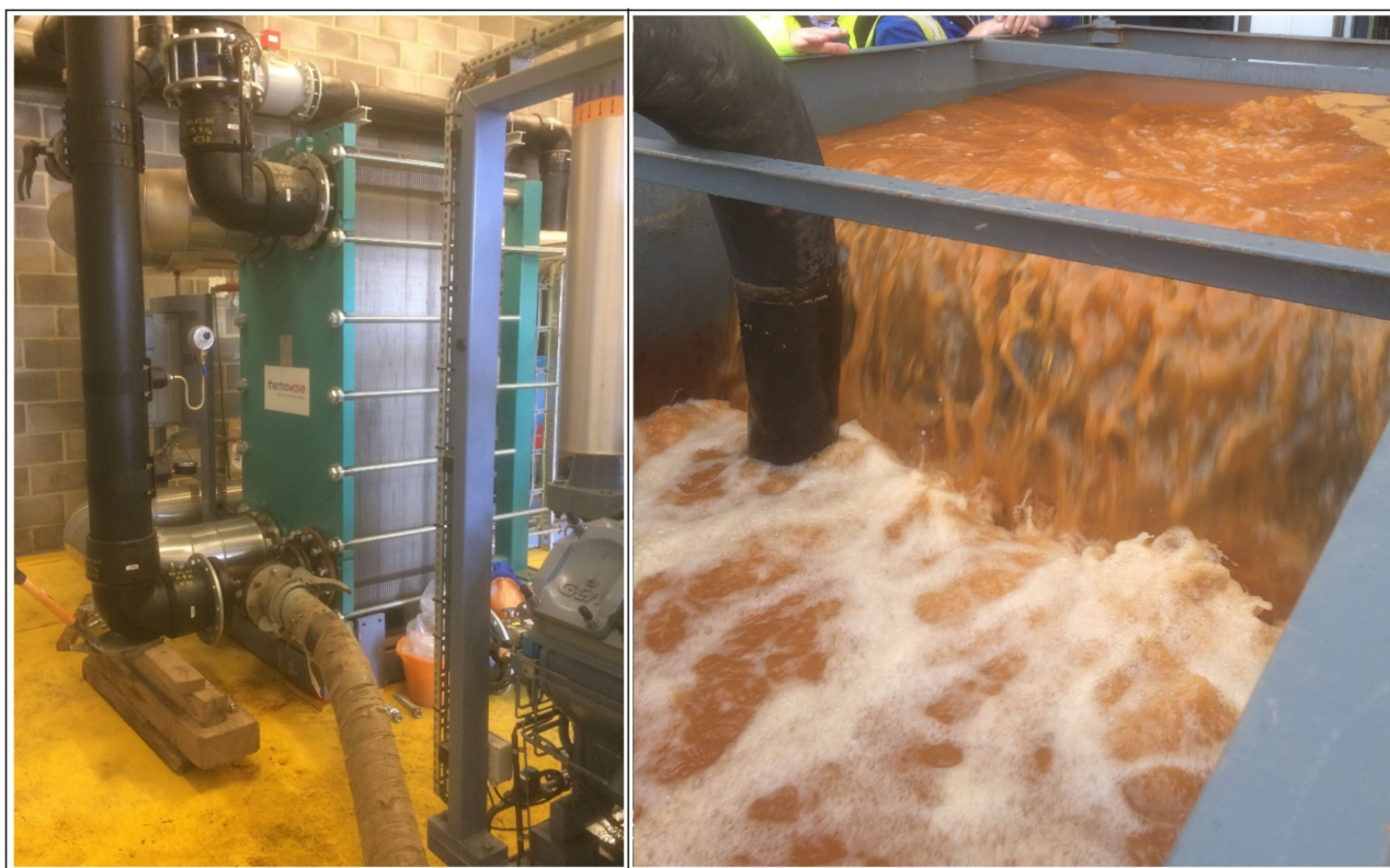
Figure 4. Periodic recirculation of citric acid solution through the plate heat exchanger at Abbotsford Road, Gateshead, UK ( left ), to remove accumulated ochre (which can be seen in the recirculation tank, ( right )). Reprinted with permission from ref. [70]. Copyright 2019 David Banks.
