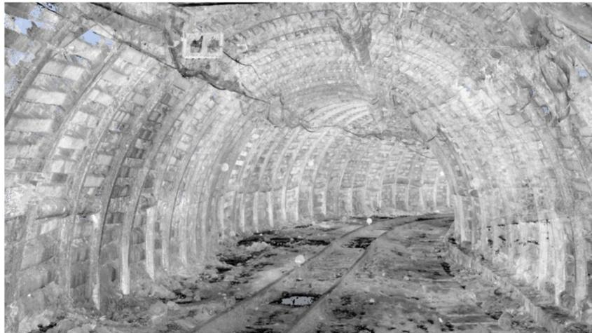
**Figure 2.** 'Inside' view of a mine gallery section before a bend—point cloud.
