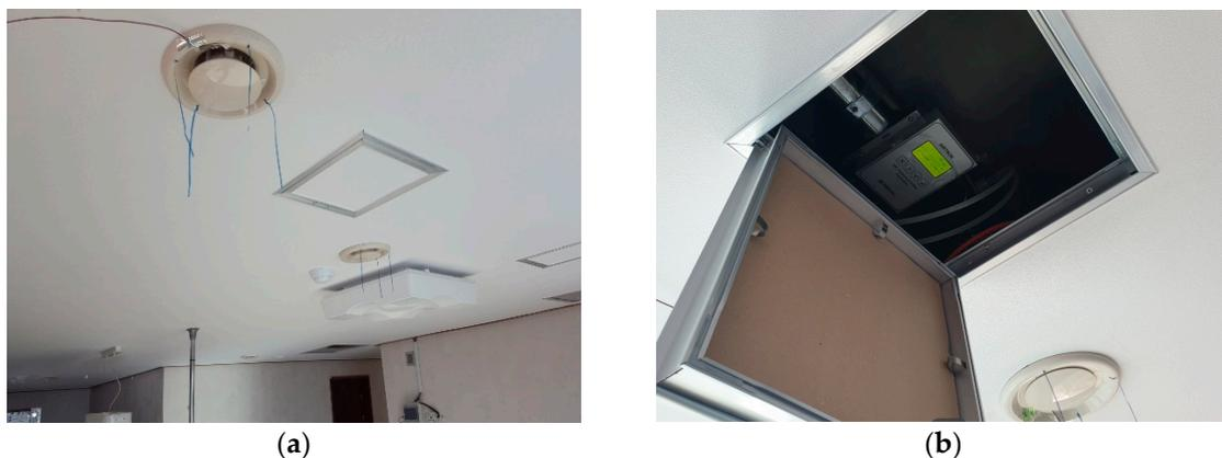
Figure 8. The diffusers (a) and transmitter installed for air flow measurement (b).
