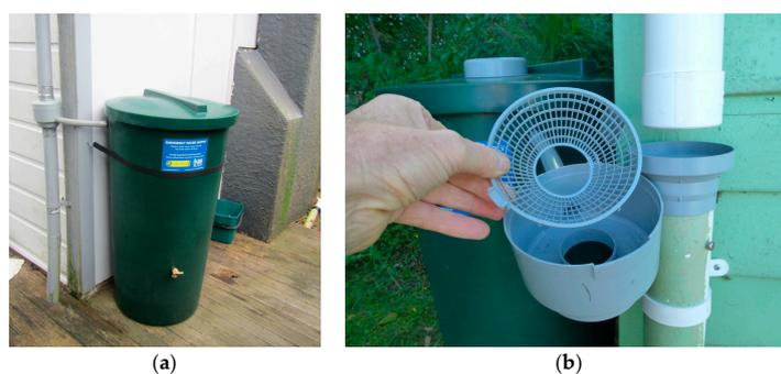
**Figure 2.** (a) WREMO emergency 200-L rainwater tank installed at Site 6; and (b) detail of diverter showing coarse screen (photo credit: Jim Cousins).
