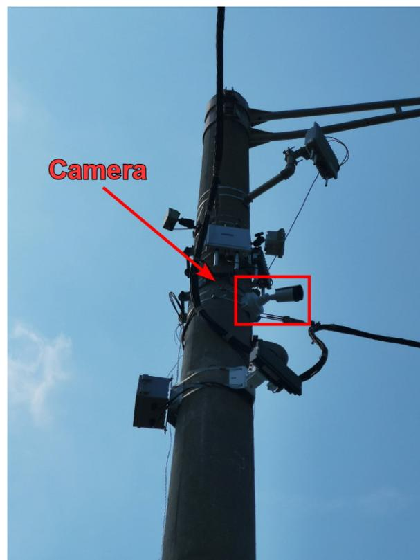
**Figure 5.** One of the network cameras installed on a traffic pole.
