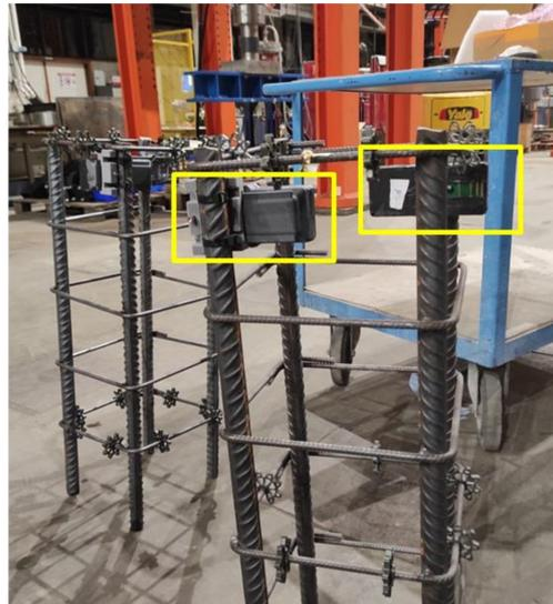
**Figure 4.** Reinforcement cages of the concrete columns before placing in the formwork. The hardware devices are highlighted.
