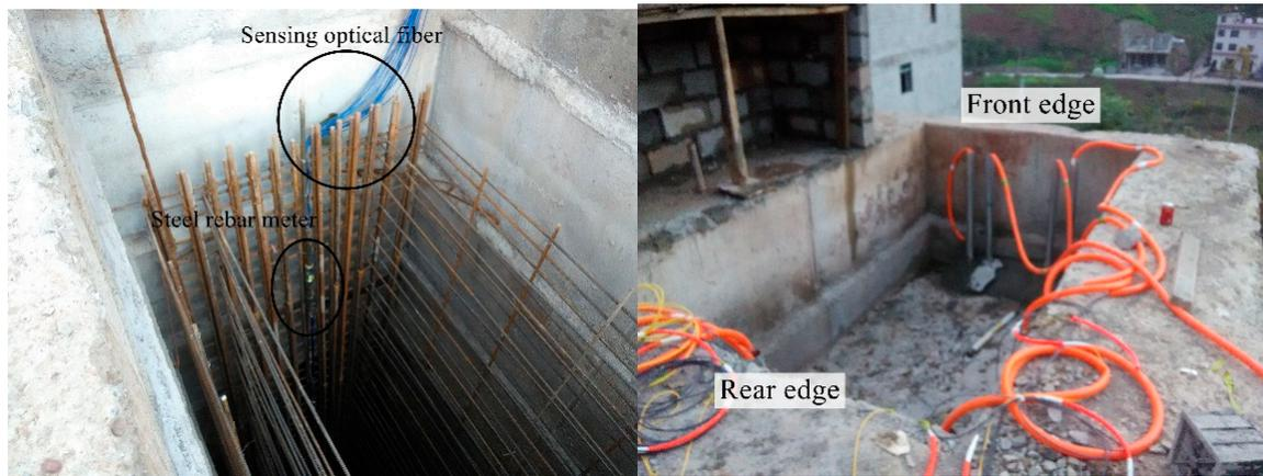
**Figure 4.** Site construction picture of the anti-slide pile.
