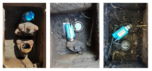
Figure 2. HWM PermaNET SU loggers deployed on hydrant control valves in different locations.
