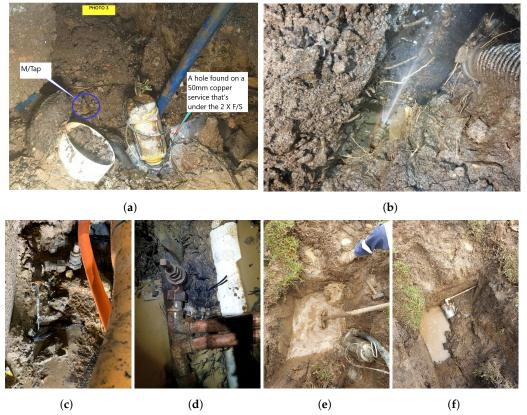
**Figure 3.** Examples of detected hidden leaks from a range of vibro-acoustic sensors and deployment areas (pictures supplied by utility field crews, taken during repairs): (**a**) Copper service leak, (**b**) Main tap leak, (**c**) Main tap leak (clamped service line), (**d**) Leak on main tap coupling piece, (**e**) leaking main tap (excavation site), and (**f**) leaking main tap repaired with full circumference pipe clamp.
