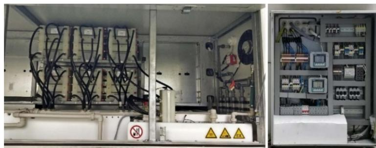
**Figure 5.** The batteries attached to the PV system including the digital meters of the monitoring panels.
