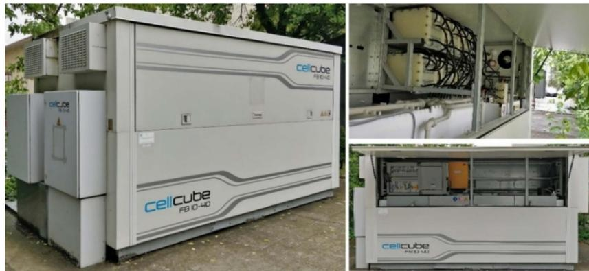
**Figure 4.** The storage unit attached to the PV system at the National Institute for Research and Development of Isotopic and Molecular Technologies, CETATEA building, Cluj-Napoca, Romania.
