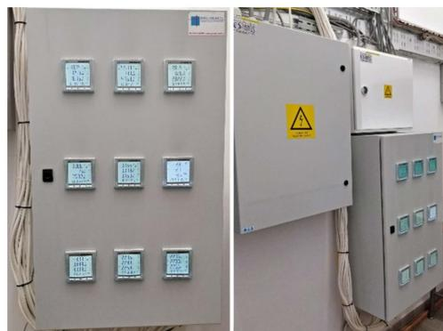
**Figure 6.** The monitoring panel of the PV system with nine digital electric meters.
