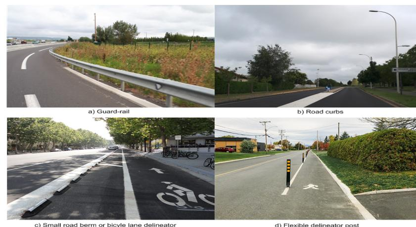
**Figure 1.** Road borders: (a) Guard rail on highway access road, (b) road curbs on urban environment, (c) small road berms used as bicycle lane delineators, and (d) multipurpose flexible delineator post.
