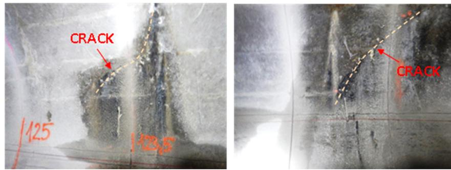
Figure 12. Examples of diagonal cracks of a collector concrete structure.
