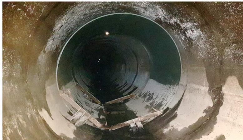
Figure 2. GRP test panel inside a collector before installation.
