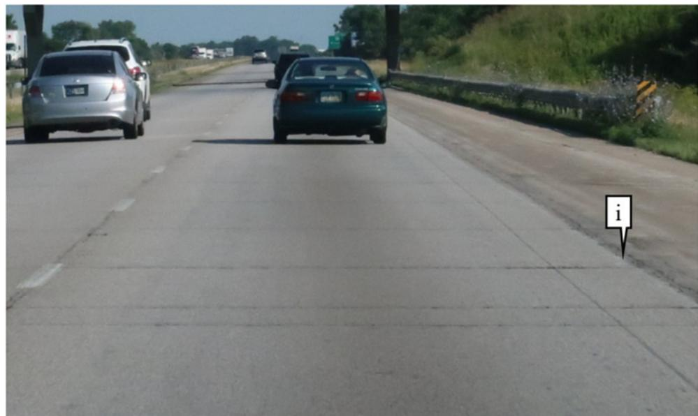
**Figure 1.** Example of deteriorated pavement marking on roadways.
