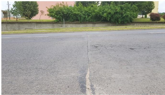
**Figure 10.** Single crack perpendicular to the direction of road (SCP), photographed from the point of view of a parked car.
